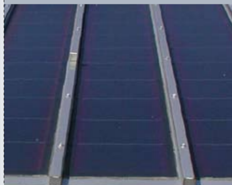
FIGURE 9: The combination of stainless steel roofing elements with integrated amorphous silicon photovoltaic modules allows for a large variety of designs.
