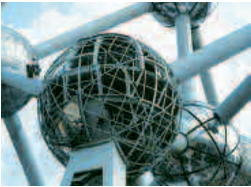
Figure 17: Fastening stainless steel outer panels to a carbon steel structure on the Atomium, Brussels
