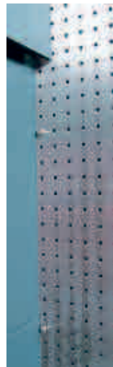
Figure 11: To prevent galvanic corrosion, only stainless steel fasteners should be used on stainless steel panels.
