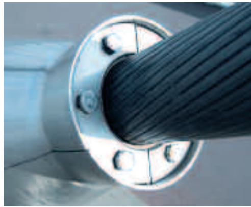
Figure 27: No galvanic corrosion will occur between different types of stainless steel, even if they do not have the same corrosion resistance.
