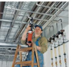
A total of 12,900 running metres of stainless steel (DN 15-150, grade 1.4401) was used in the accident and emergency clinic in Murnau.
