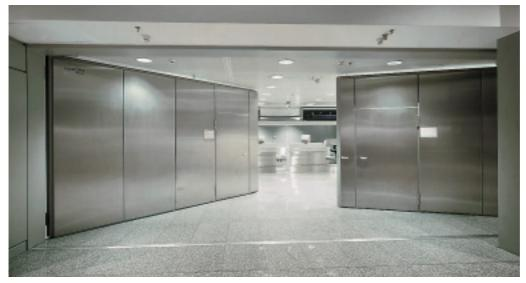
The double fire gates in Terminal 2 at Frankfurt Airport are made entirely in stainless steel, and meet fire resistance standard T90. A built-in escape door offers a means of exit even when the gates are closed.
