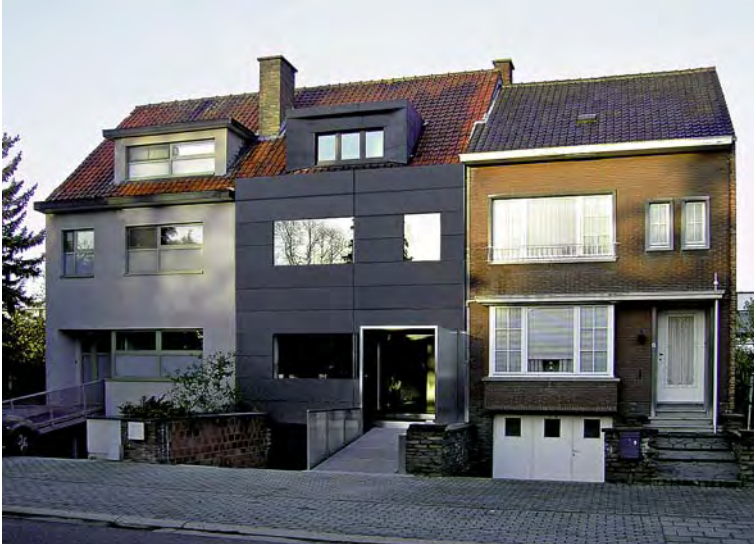
Part of the new stainless steel entrance porch projects from the insulated, fibrated-concrete façade.
