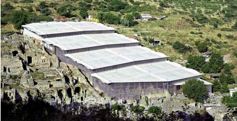
The shelter for Terrace House 2 covers over 4,000 m 2 of space. Tracing the line of the slope, it blends well into the ancient site.
