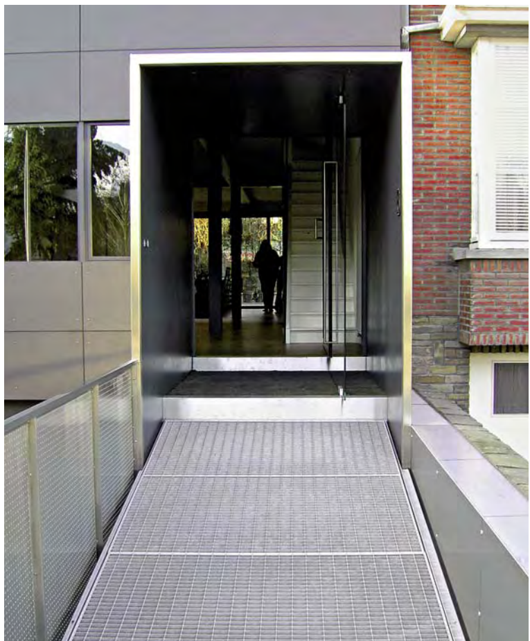
A ramp of galvanized metal grating bridges the height difference between the street and the front door.
