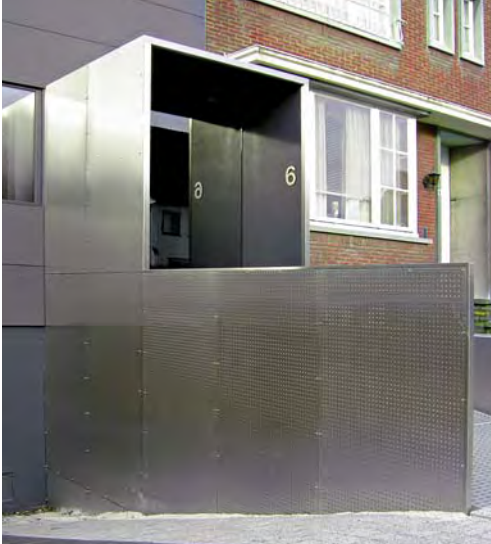
The entrance porch was built to a design worked out with a skilled metal-worker on site.
