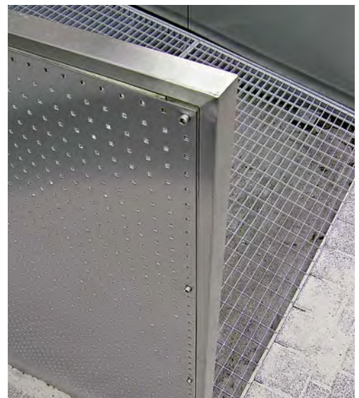
The parapets of the small ramp are clad with perforated and smooth stainless steel sheet with a ground finish.
