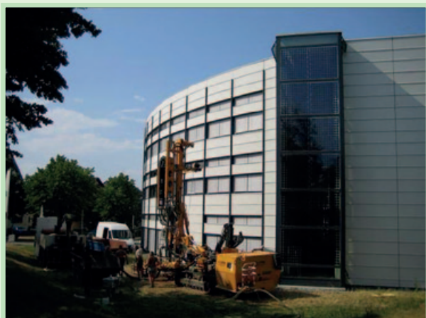
80 metre deep holes were drilled into the ground to accommodate the geothermal probes
