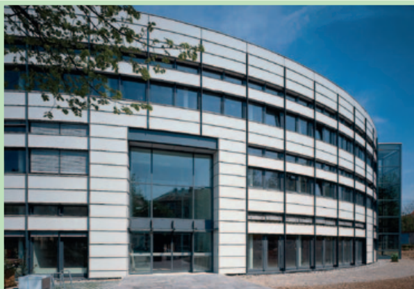
Fraunhofer ISE was selected as the location for a large-scale test of solar cooling
