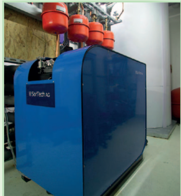
The adsorption machine is essentially maintenance-free throughout its entire useful life
