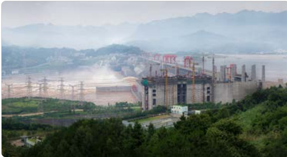
The Three Gorges Dam in China
