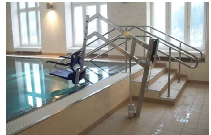
Indoor swimming pools are among the most corrosive environments and require corrosion-resistant materials.
