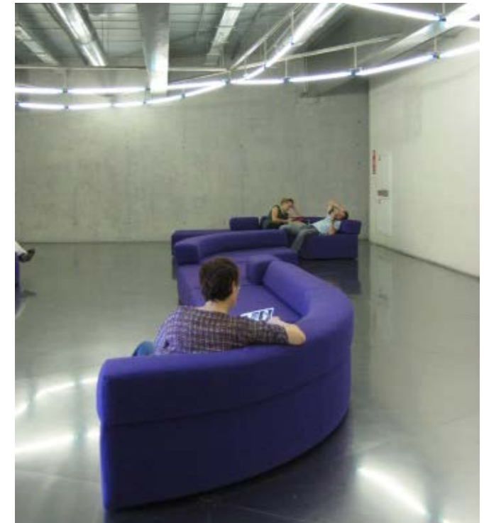
Despite its reflective character, stainless steel sheet can be made slip-resistant, as shown in the Caixa Forum exhibition hall in Madrid, Spain.
