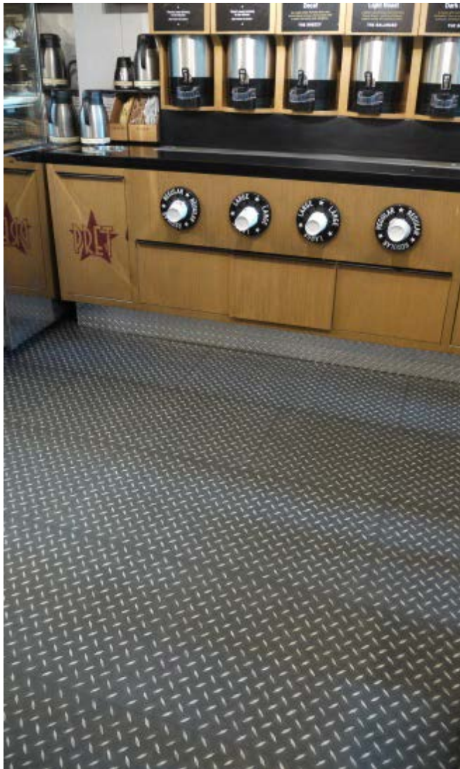
Stainless steel tread plate in a coffee shop in New York. Photo: Euro Inox, Brussels, Belgium
