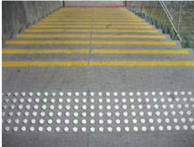
Tactile floor guidance systems in stainless steel are durable and attractive. Photos: Euro Inox, Brussels, Belgium
