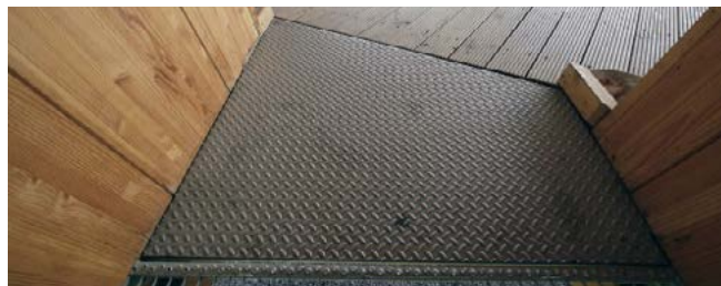
Stainless steel flooring in a visitors centre, Koblenz, Germany. Photo: Euro Inox, Brussels, Belgium
