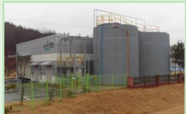
Figure 13: Bousung Biogas Plant 12
