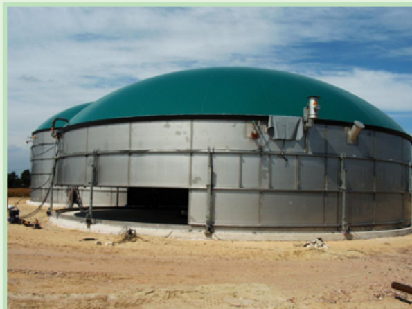
Figure 5: Construction of a stainless steel digester tank 4
