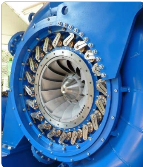
Francis micro hydro turbine in Kvernerud, Norway Power: 507kW Head: 59m Flow: 1.2m 3 /s Refurbishment in 2008 of a 1917 plant Top: complete installation with turbine (blue) and generator (red) Left: open view of turbine outlet and gates for flow control Pictures courtesy of Hydrohrom s.r.o. Czech Republik
