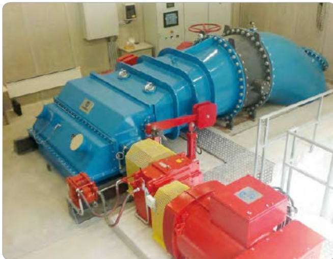
Left: Crossflow turbine Picture from Ossberger Right: Close-up of a stainless steel rotor Picture from Irem spa
