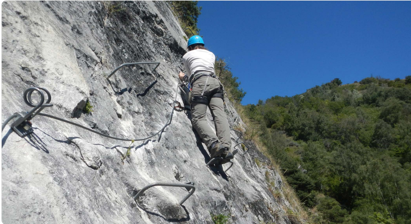
EN 1.4301 (AISI 304) rebar rung to be anchored into the rock.
