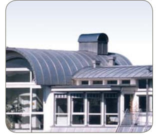
430Ti (standing seam technique), Ugine & Alz, 호주
