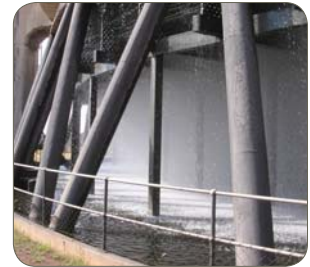
발전소 (POWER GENERATION)
