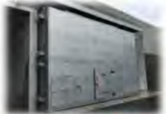
Koishihama Gate (SUS821L1) 小石滨水闸 (SUS821L1)
