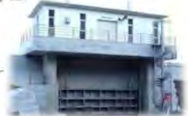
Kosode Gate (SUS821L1) 小袖水闸 (SUS821L1)
