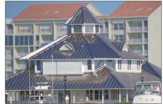
Stainless steel roofing system, more than 50 years
