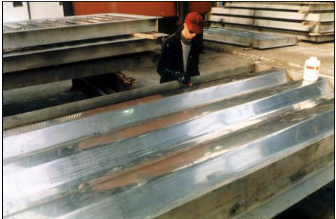
A trapezoidal blast resistant wall being fabricated for the topsides of an offshore platform
