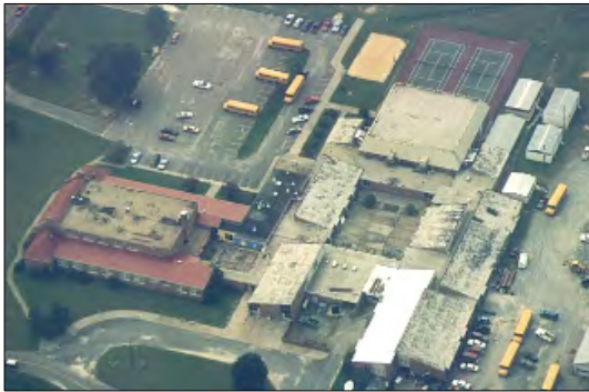
Conventional roofing systems, ~30 years
