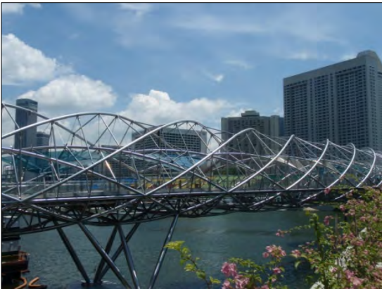
Helix Bridge, Singapore, 2011
