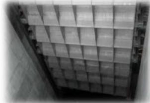
Kanogawa Dam (SUS821L1)
