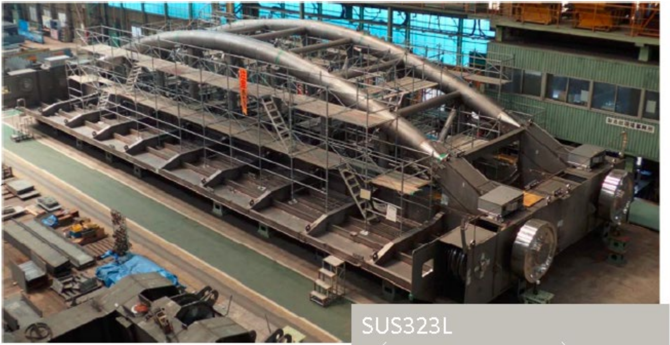
A view of the gate being built
