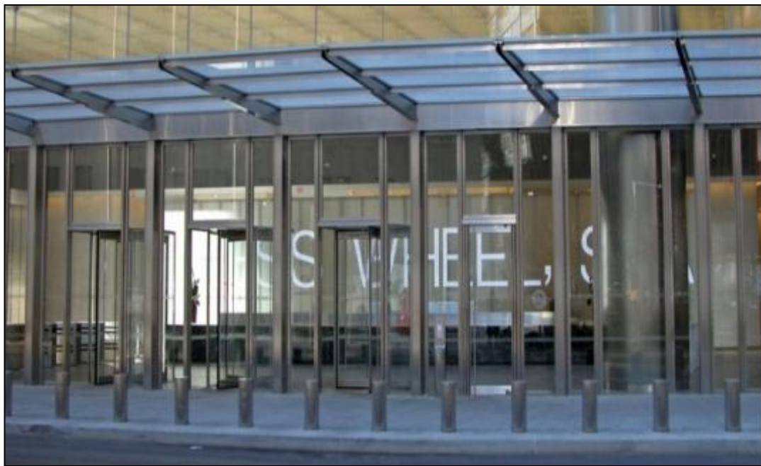
Blast resistant columns in entrance canopy, Seven World Trade Centre, New York
