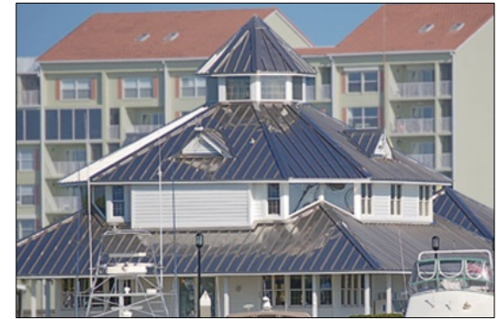
Stainless steel roofing system, more than 50 years
