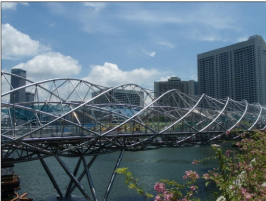
Helix Bridge, Singapore, 2011
