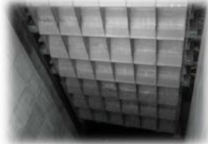
Kanogawa Dam (SUS821L1)
