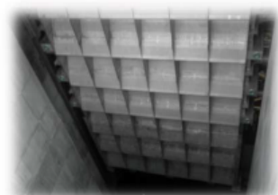
Kanogawa Dam (SUS821L1)
