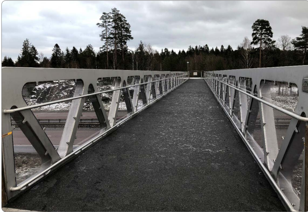
The bridge installed over E4 in Södertälje south of Stockholm, Sweden.
