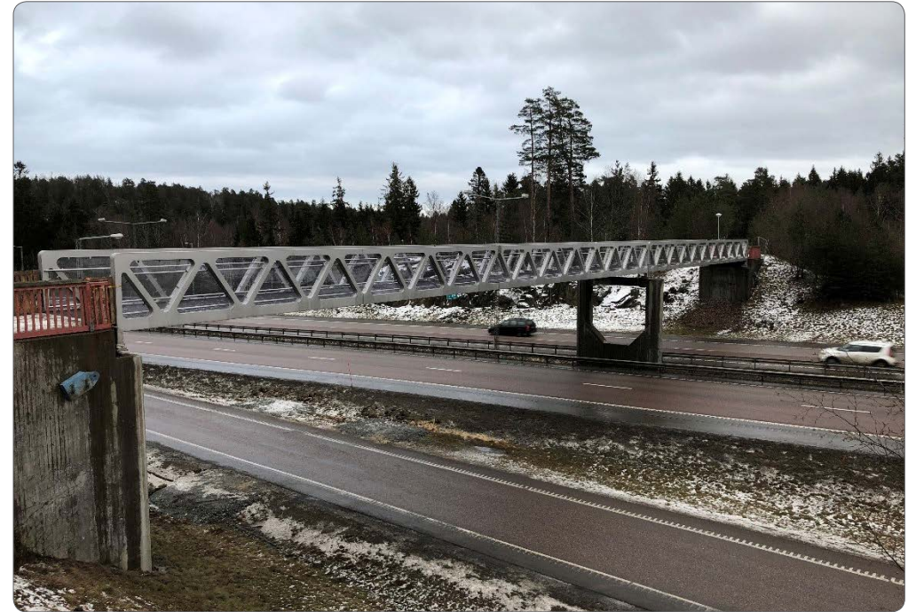
The bridge installed over E4 in Södertälje south of Stockholm, Sweden.
