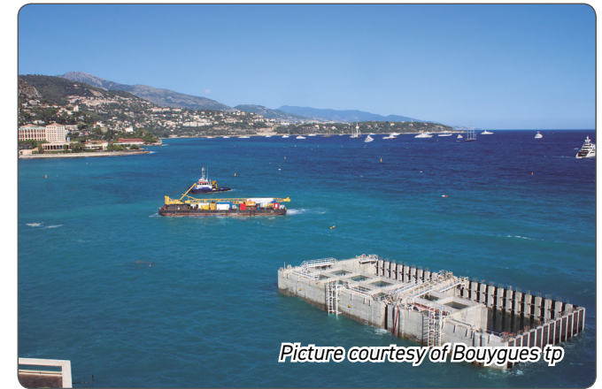
Picture 5: Caisson being positioned in the sea
