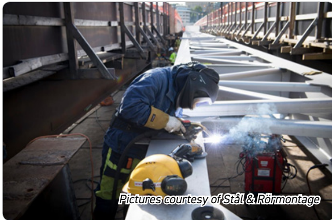
Picture 3: Installation of new structure in grade Forta LDX 2404
