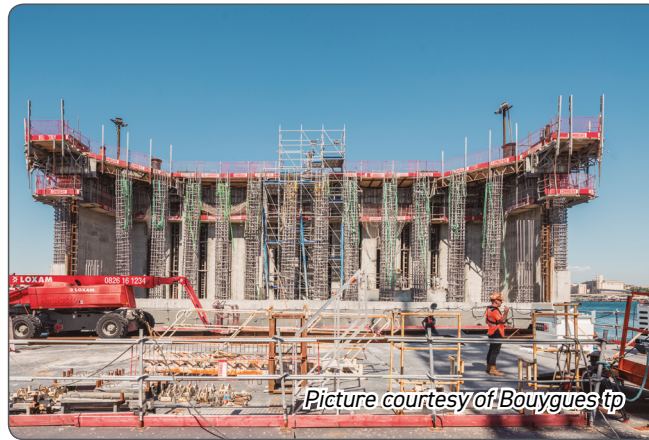
Picture 4: inside view of an unfinished caisson
