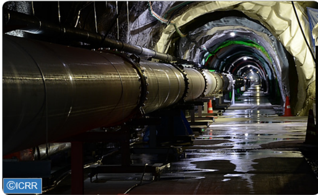
Photo 2: Ultra-high vacuum stainless steel duct of 3,000m in length, as the laser path in the interferometer
