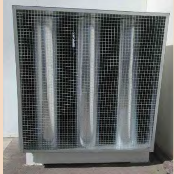
Example of a sound attenuator installed by Böllinghaus
