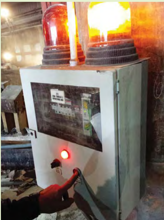
Workers can activate the new warning lights at a press of a button
