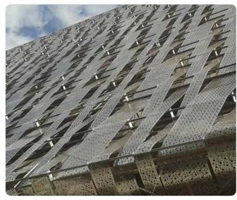
Environment: urban outdoor Fabrication process: perforation Grade and finish: 444, 2B
