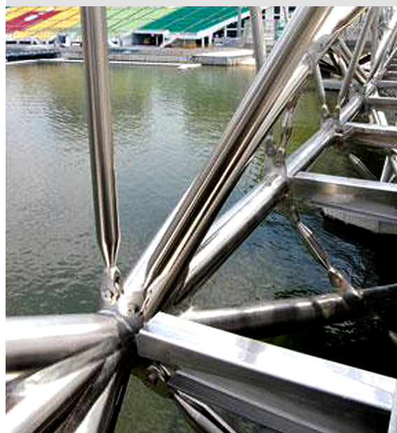
Figure 5: Connection included welded and pinned joints (Photo: Arup)
