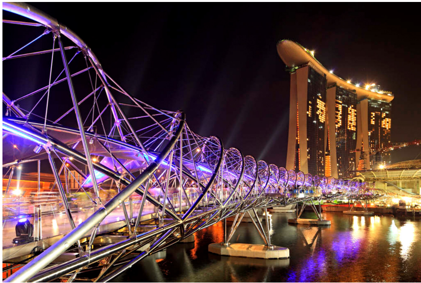
Figure 1: General view of the Helix Bridge
