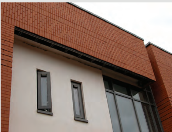
Figure 5: Construction of vertically stack bonded brickwork held up by masonry support system
