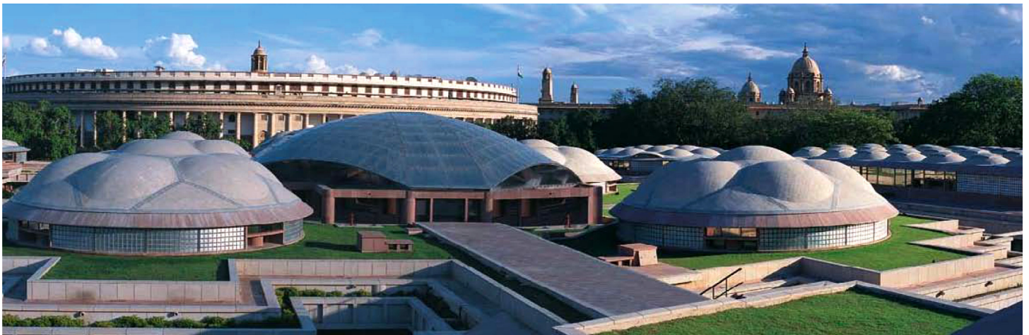
Figure 1: General view of the domes of the New Delhi Parliament Library
