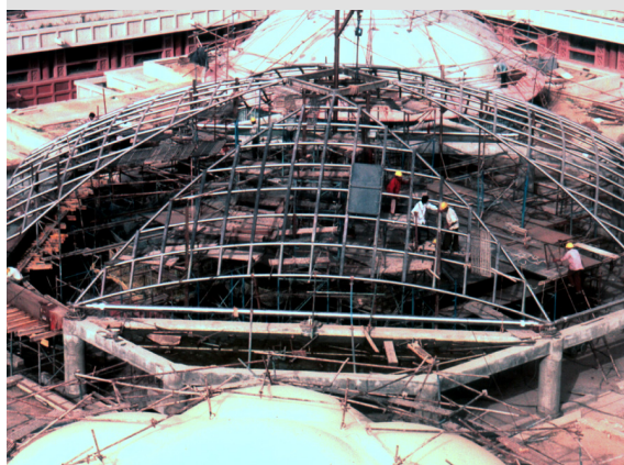
Figure 8: Erection of the focal dome
