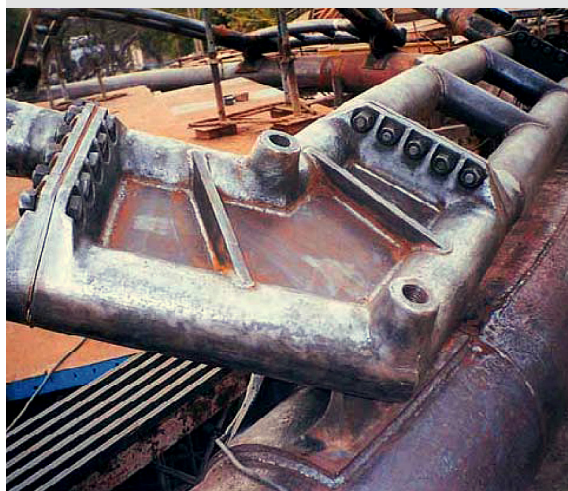
Figure 9: Steel members assembled on site during construction
