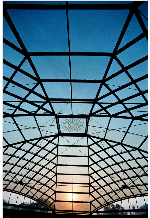
Figure 3: View of the stainless steel and glass central focal dome
