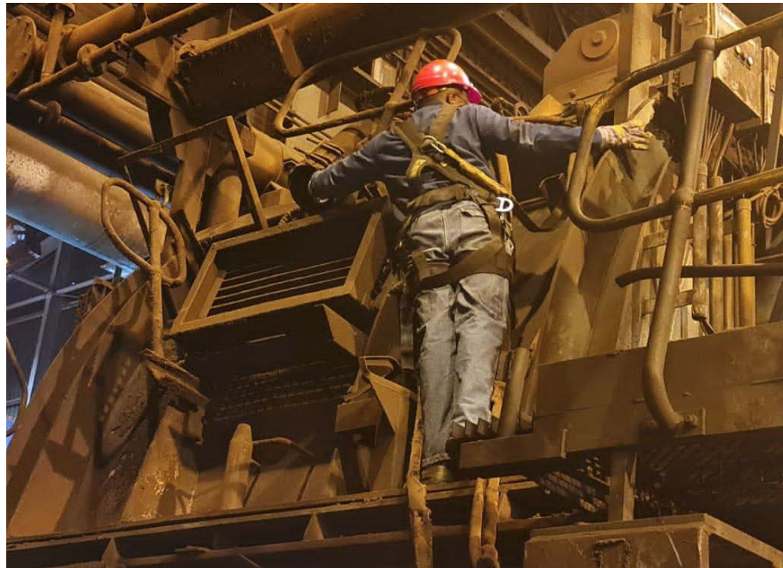
Picture 1 - Old method (harness and stepping off safe platform)
