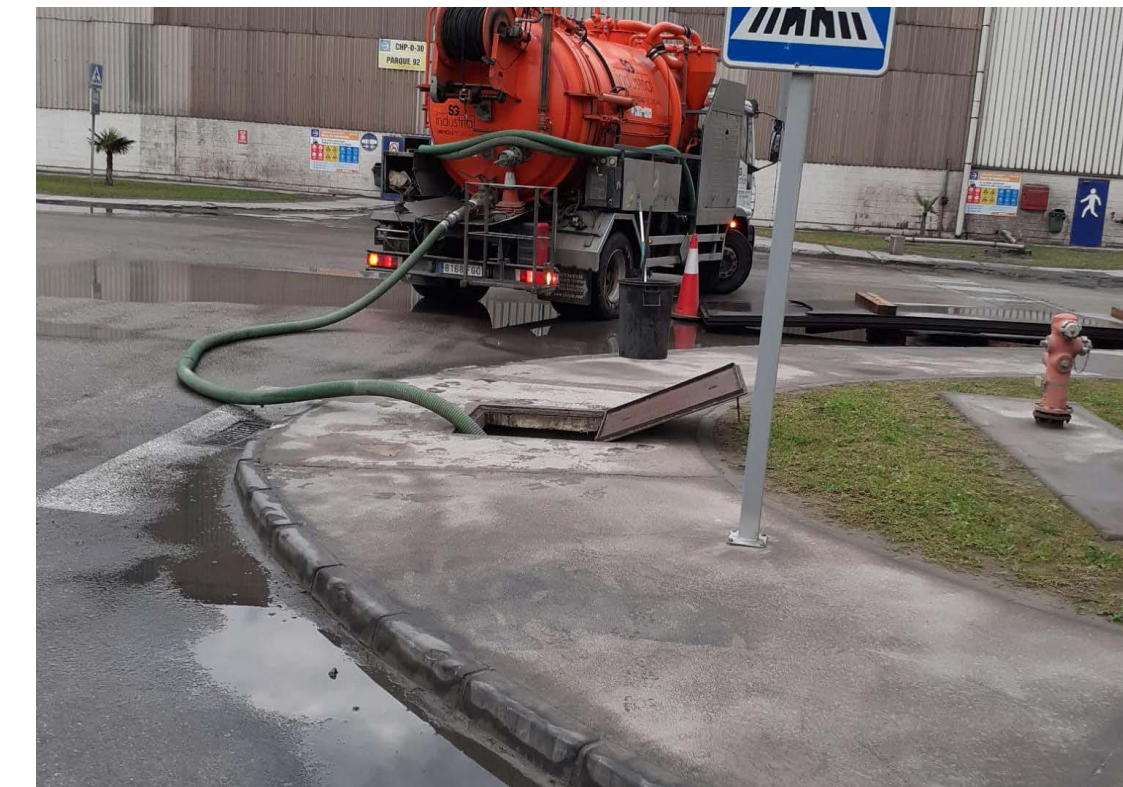
Image 1. Wasted water is refilled to a tanker truck with own pump from gutter.
