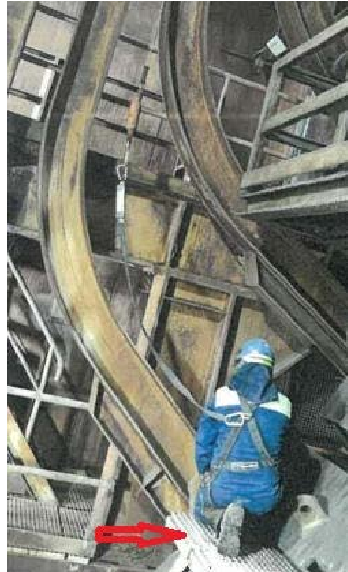
Figure 4: operator on the new platform
