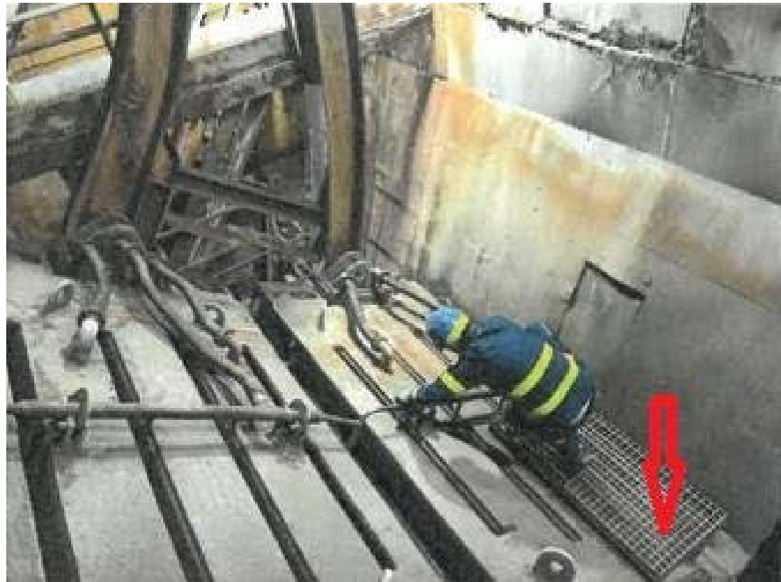
Figure 3: operator on the new platform
