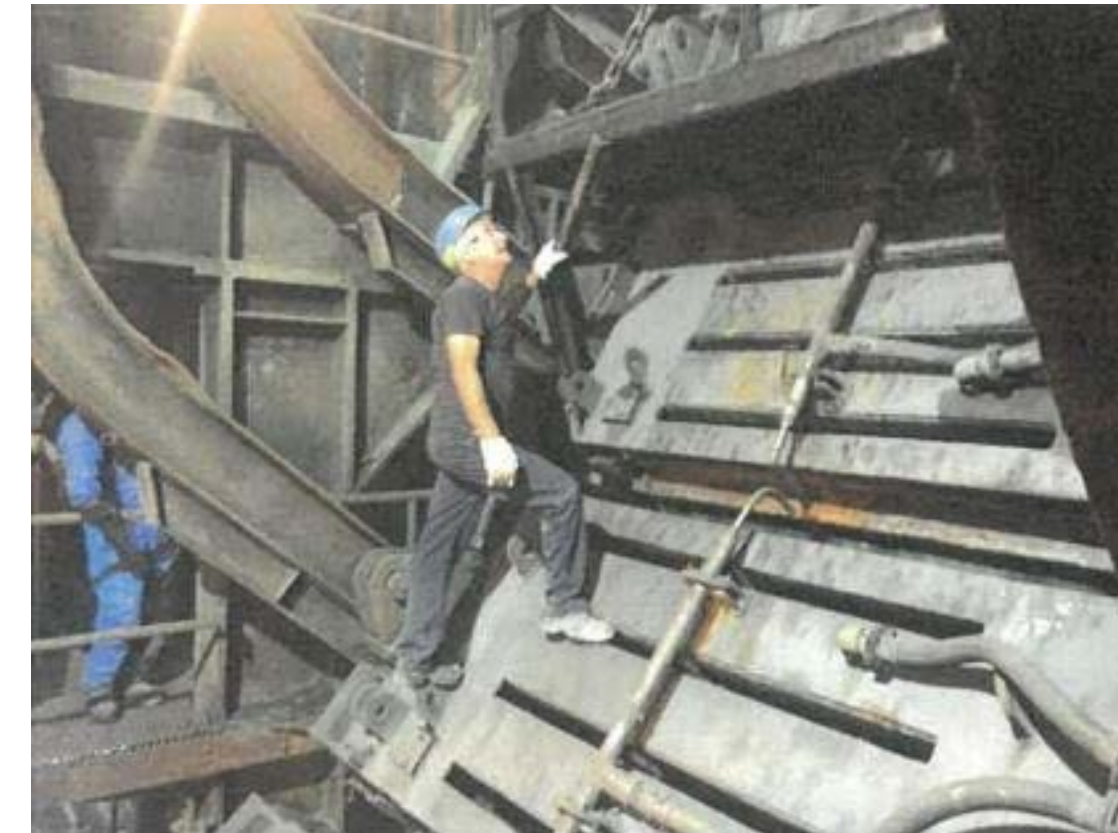
Figure 1: operator on the continuous casting segment
