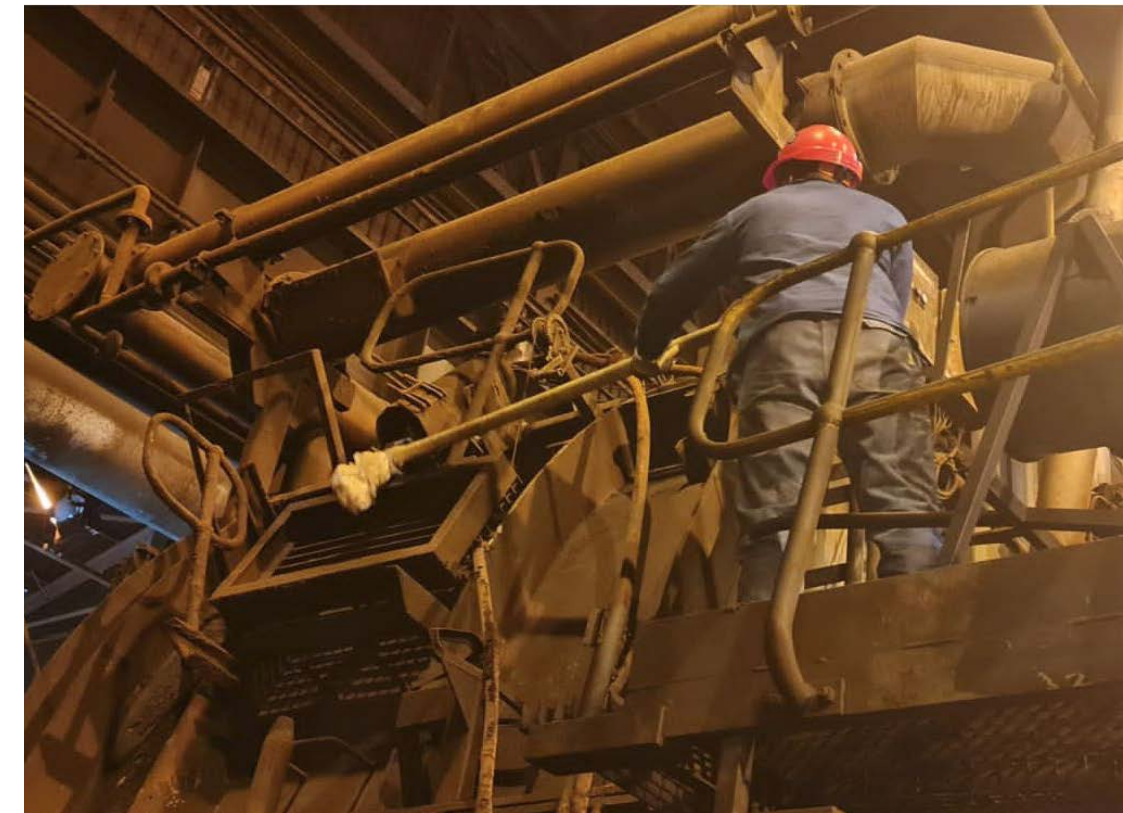
Picture 2 - New method with tool (standing on safe platform)
