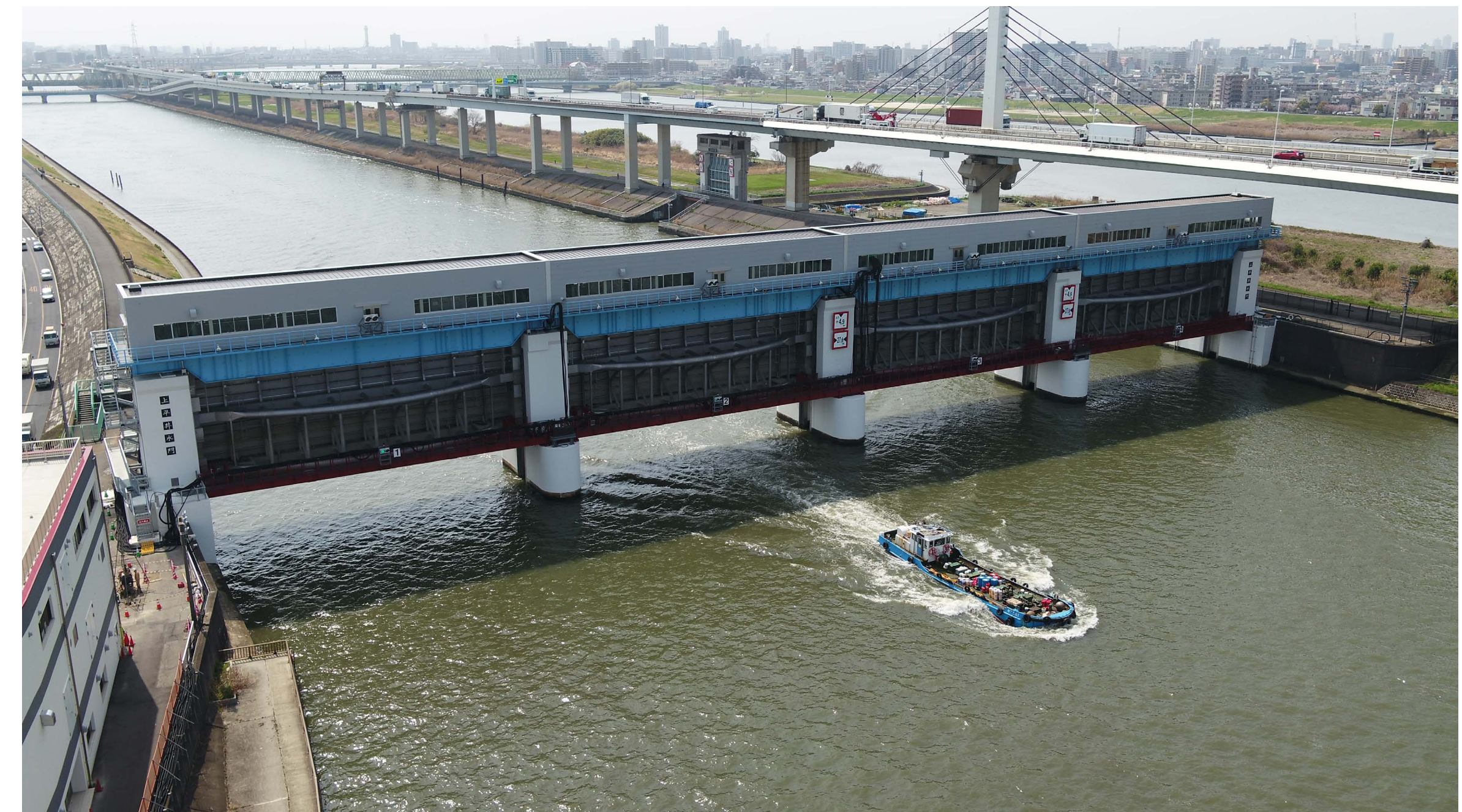
Kamihirai Flood Gate (Full view of flood gate(from upper stream side))
